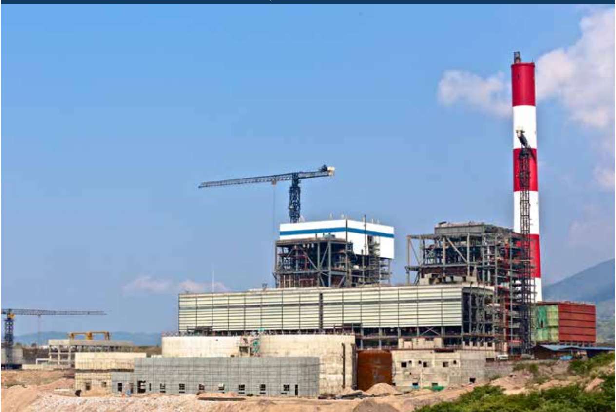
300 MW POWER PLANT UNDER CONSTRUCTION AT MAAMBA, ZAMBIA
